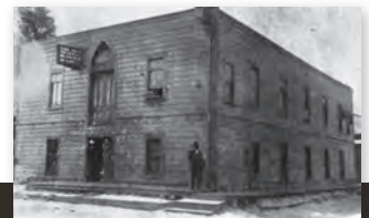
1906 Outpouring of Holy Spirit on Azusa Street in Los Angeles
